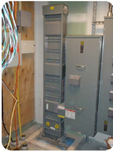
Figure 3: Bus Duct
