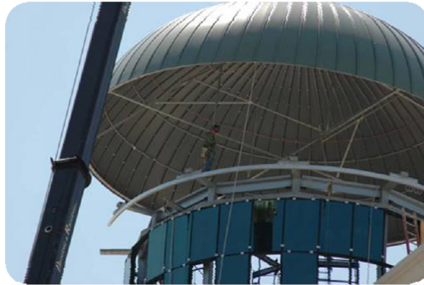
Figure 2: Placing Cupola Dome
